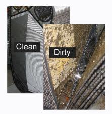
Heat exchangers are often utilized as a source for removing heat from industrial cooling processes. Small orifices can become plugged quickly with debris leading to reduced heat transfer, lower efficiencies, increased head pressures and higher maintenance costs.
