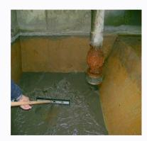
Over time sumps, pits and basins collect solids. Manually removing these solids can increase liablility and maintenance costs.
