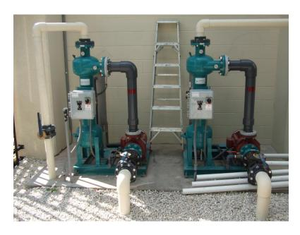
**Status:** Two Puroflux PF-64-050-AP hydrocyclone solids separator packages with automated purge valves were installed into the water processing system and effectively purge the collected solids down the drain and out of the way of the treatment chemicals as intended.
